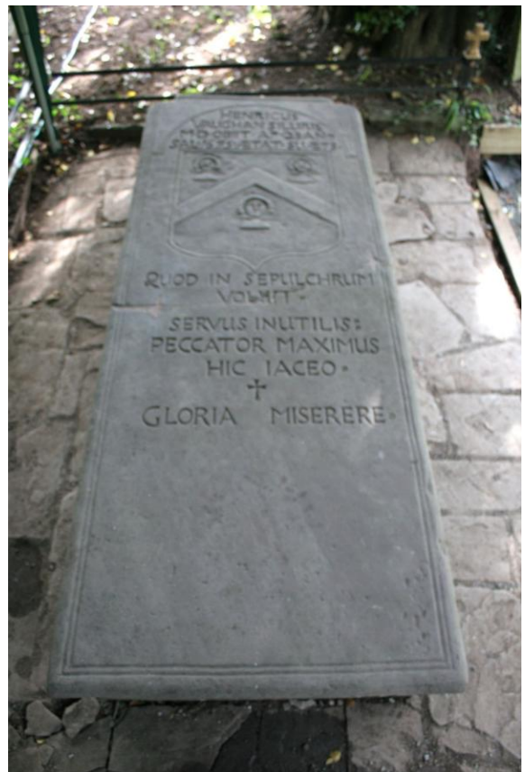
General views of the top incised inscription slab during cleaning on the left and with all treatments completed on the right. Note the laminar structure of the stone slab is much more pronounced after cleaning, with light and dark banding. Note how uniformly colonized the un-cleaned upper section is, this will happen again relatively quickly, causing the new alkaline surface of the hydraulic lime filling medium to blend in with adjacent sandstone surfaces.
