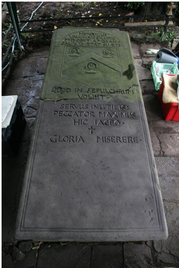
General views of the top incised inscription slab during cleaning on the left and with all treatments completed on the right. Note the laminar structure of the stone slab is much more pronounced after cleaning, with light and dark banding. Note how uniformly colonized the un-cleaned upper section is, this will happen again relatively quickly, causing the new alkaline surface of the hydraulic lime filling medium to blend in with adjacent sandstone surfaces.
