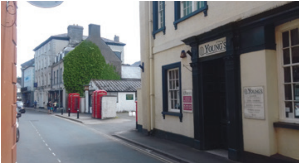
Figure 14. The gap in St Mary's Street, Brecon, created by the demolition of the Mansion House (the surviving kitchen wing is to the right).
