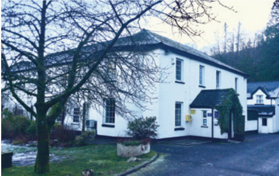
Figure 13. The surviving portion of the Morgans' Shooting Lodge at Nant Ddu, showing the Western curved bay which accommodated the drawing room on the ground floor and Lord Tredegar's bedroom on the first floor.
