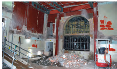
Figure 3. The Assize Court Hall after demolition of the waffle slab.
