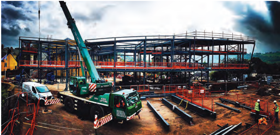
Figure 1. Y Gaer in September 2017 showing the erection of the steel frame.
