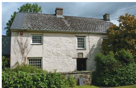
Figure 33. Aberhoyw: front elevation with 1726 date-stone.
