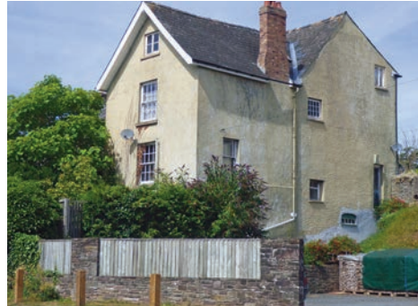
Figure 10. The site of Mount Street station.
