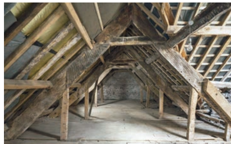
Figure 29. Old Gwernyfed: reused roof-trusses.
