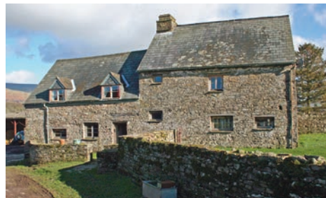
Figure 20. Pen-y-bryn (Llangatwg): front elevation with stepped roof line.
