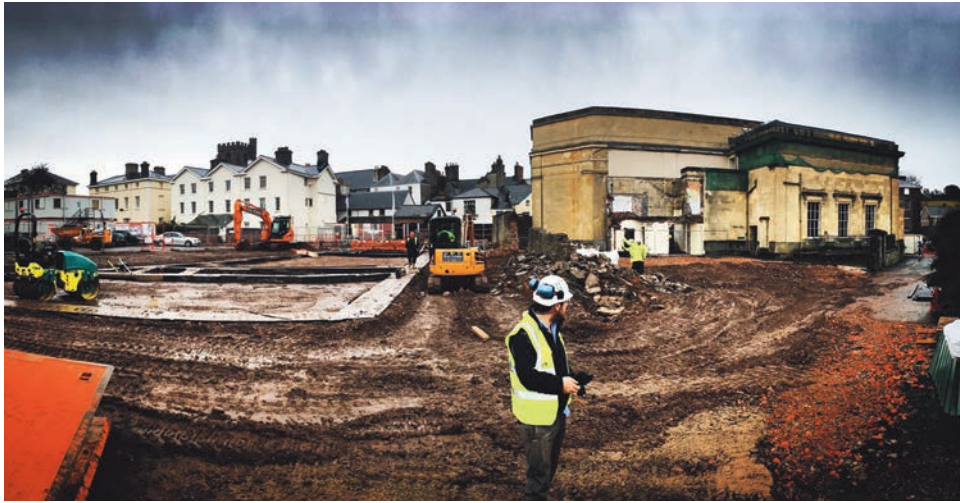
Figure 1. The foundations for the new atrium and library.
