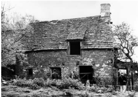
Figure 1. Work in progress on the Buildings of Breconshire at Penyrheol Cwm Du.
