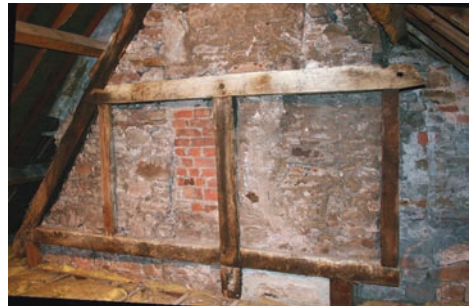
Figure 6. Priory House, Brecon: thirteenth-century roof-truss in the old Deanery.
