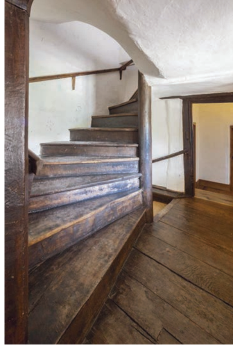
Figure 25. Old Gwernyfed: a mast stair.
