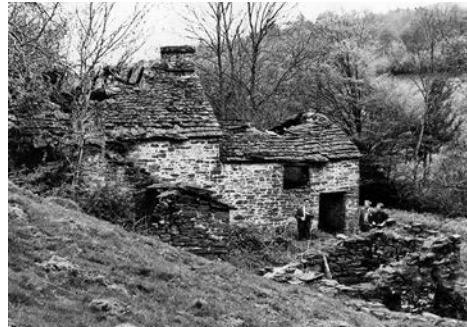
Figure 2. Work in progress on the Buildings of Breconshire at Tyn y Cwm, Llanbedr.
