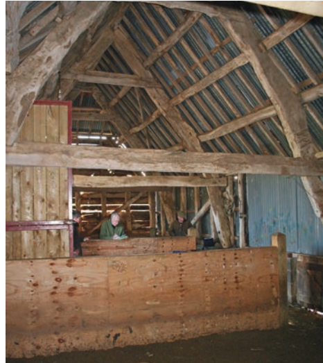
Figure 24. Maes-llech (Llanlleonfell): cruck-trussed and timber-walled barn.
