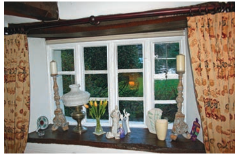
Figure 17. The Elms (Talgarth): parlour window with ovolo moulding.
