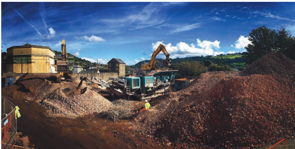
Figure 1. Demolition at the site of the Brecon Cultural Hub during September.
