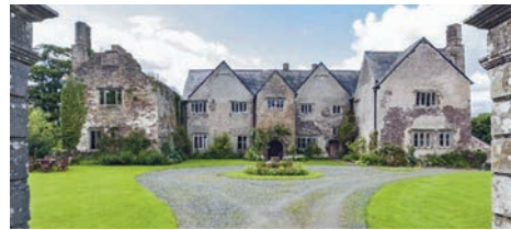
Figure 16. Old Gwernyfed: front elevation with ruined parlour wing.
