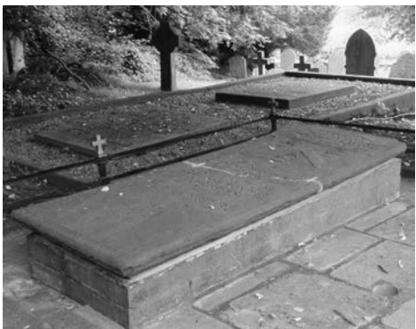
Fig. 2 (a) Restored grave of Henry Vaughan and newly laid flagstones July 2014. The mortar in the gravestone will ‘weather’ with time.
