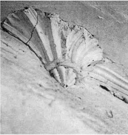
Plate 3 Plasterwork in the Great Chambers: frieze and springer of ribbing.
