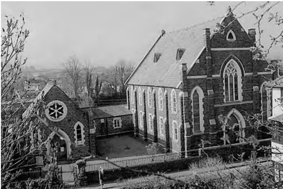
Plate 1 Kensington Baptist Chapel (1880–2010) showing the 1885 extension of 3 classrooms
