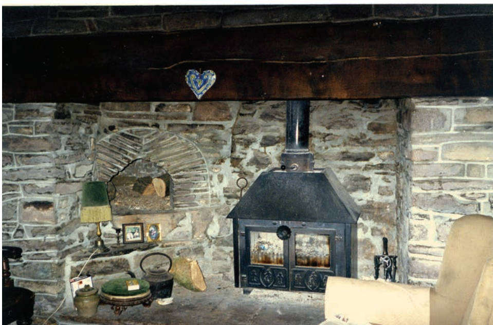
Fig. 9b Hendreforwydd, Llangattock, interior, 1997. Top: post-and-panel partition in the hall. Bottom: fireplace with bread oven.
