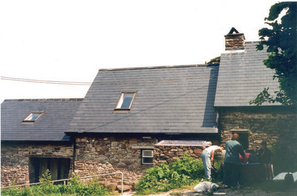
Fig. 10 Fedw, Hillside, Llangattock. Top: the longhouse, 1964. Photograph from Jones and Smith. Bottom; the longhouse converted into holiday accommodation for a Bristol youth club, 1997.
