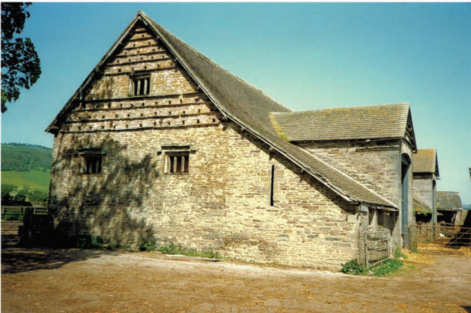
Fig. 14a Dderw, Pipton. 1997. Top: farm yard. Bottom: large barn, dated '1687, porches and aisles added 1854'.
