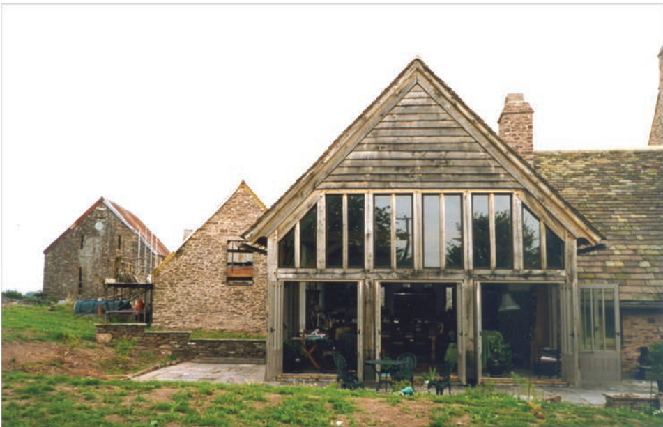
Fig. 15a Tredwstan Court. 1997. Late 17c. gentry house in course of restoration.
