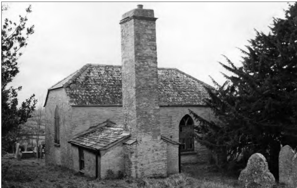
Figure 4 Penyrheol Chapel c.2001. Rear and side elevations from the east showing the former vestry, now a kitchen.
