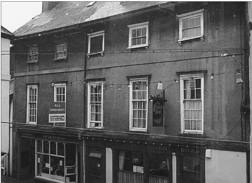
Plate 1 Bell Inn showing first floor of Great Room (front view).
