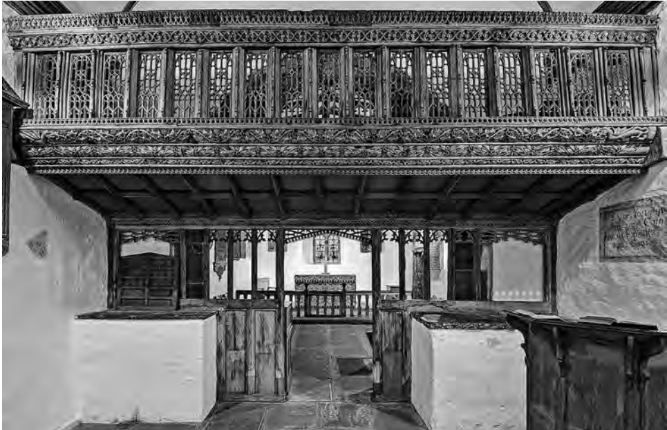
Figure 13. Photograph of Patricio Church roof screen.
